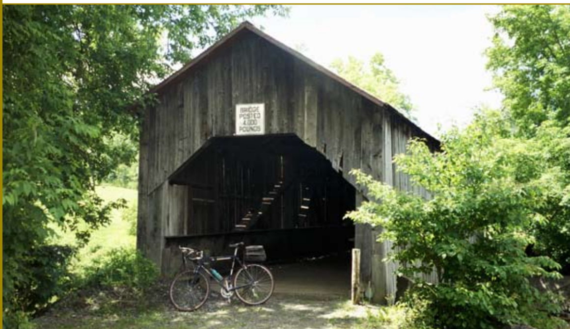
East Fairfield Bridge, East Fairfield, VT, courtesy Lou Bresee.
